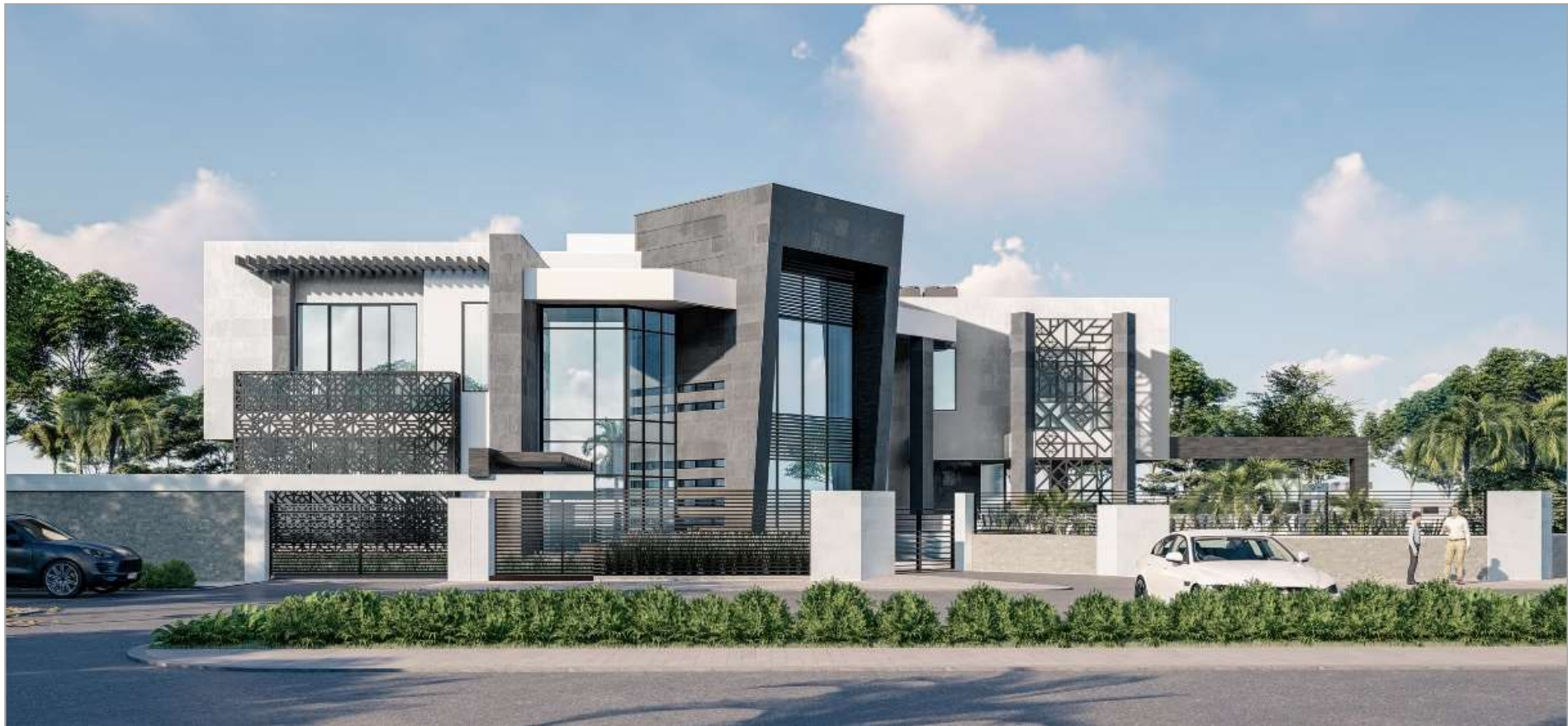
Residential Villa at Um Suqeim, Dubai
